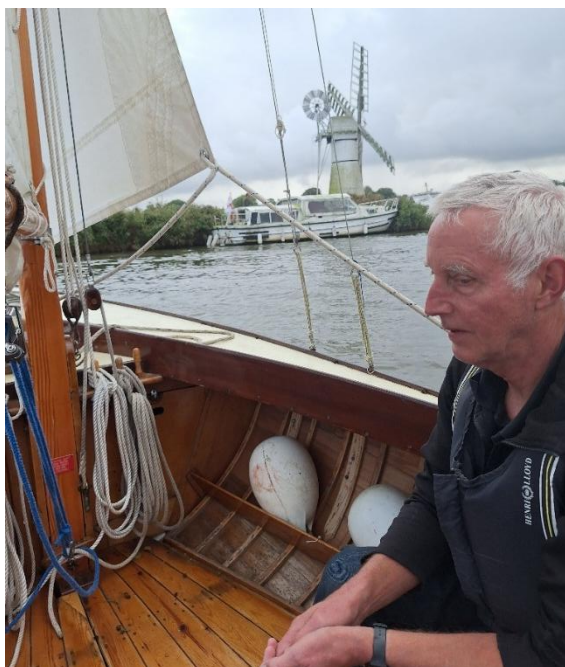
A view of one of the wind driven pumping stations
